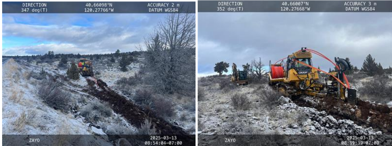
Figure 7. View of typical plow operations in Central Area (Lassen County).
