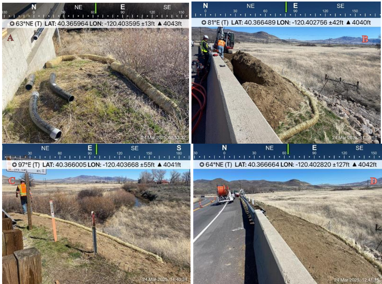
Figure 8. Examples of ground disturbing activities Bridge Tie-ins in Lassen County for March 2025: (A) BMP installs prior to earthwork at L-71.2; (B) excavation spoils from L-71.2; (C) Tie-in restoration at L-71.2; (D) completed and backfilled and graded excavation at L-71.2.
