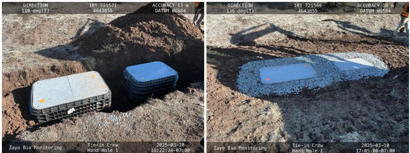
Figure 6. View of typical handhole operations in Northern Area (Modoc County).
