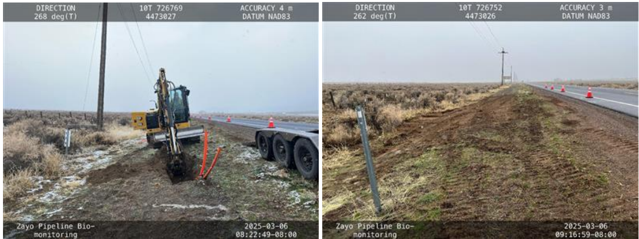
Figure 5. View of typical tie-in operations in Southern Area (Lassen County).
